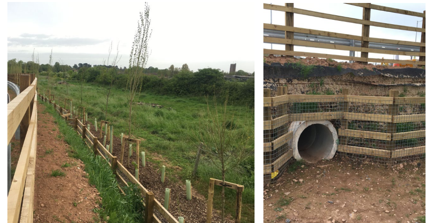
Tree planting, receptor area and badger tunnel.
