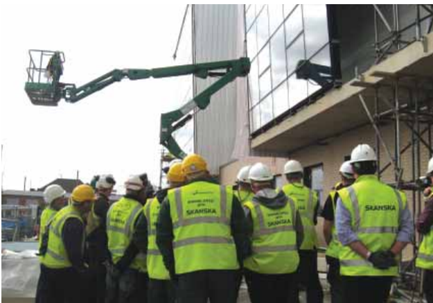
Supply Chain Staff undertaking MEWP familiarisation and rescue.
