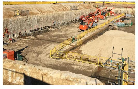
Diaphragm walling refers to the in-situ construction of vertical walls by means of deep trench excavations. Stability of the excavation is maintained by the use of a drilling fluid, usually a bentonite suspension.
