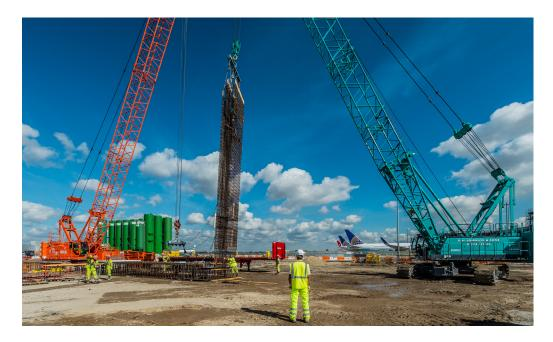
Management of the bentonite or alternative drilling fluid requires controlled use of specialist desanding, desilting and centrifuge equipment. Unit capacities range from 100 to 500m<sup>3</sup>/hour.
