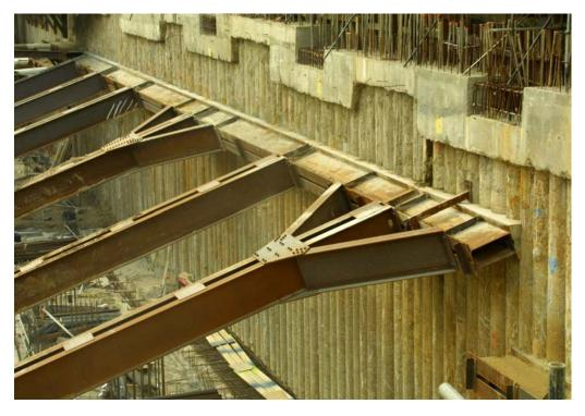
Large and small diameter bored cast-in-place piles are often used to construct efficient and economic temporary or permanent retaining walls. These walls are suitable for deep basements, underpasses, tunnel portals and other underground structures particularly where working space is limited and adjacent structures require support. They minimise bulk excavation and help to control ground movements and groundwater ingress.
