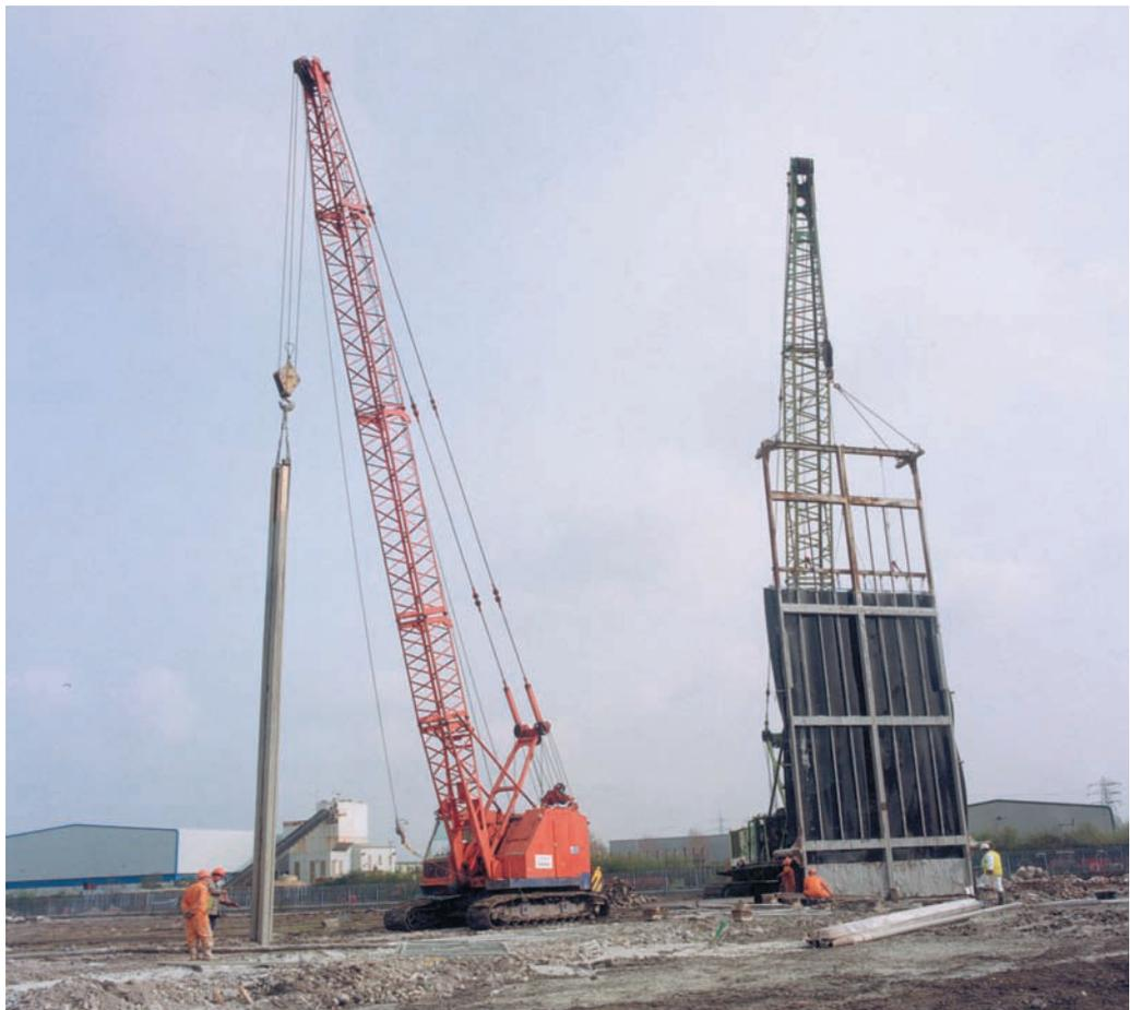
Slurry Trench Cut-off Walls provide barriers to the movement of gas and/or leachates from contaminated sites and refuse dumps etc. They can also be used to control the movement of ground water, where required.
